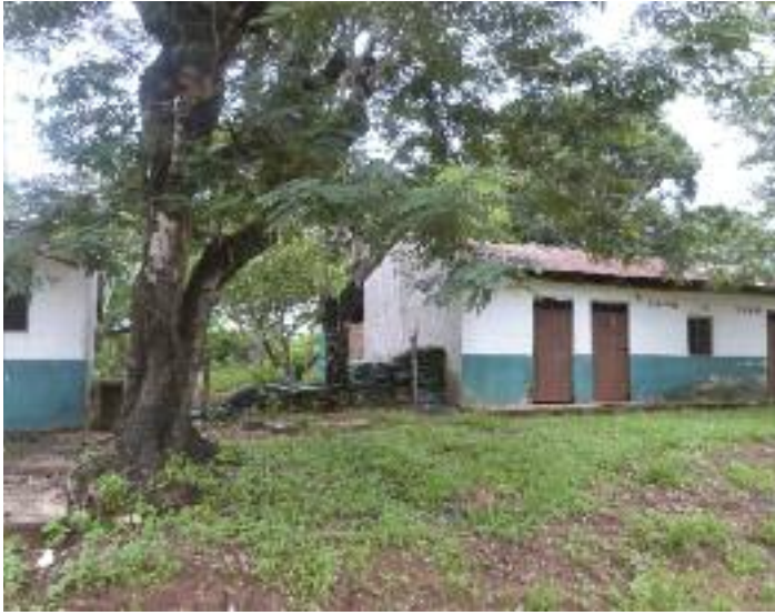
Abandoned police station in El Porvenir
