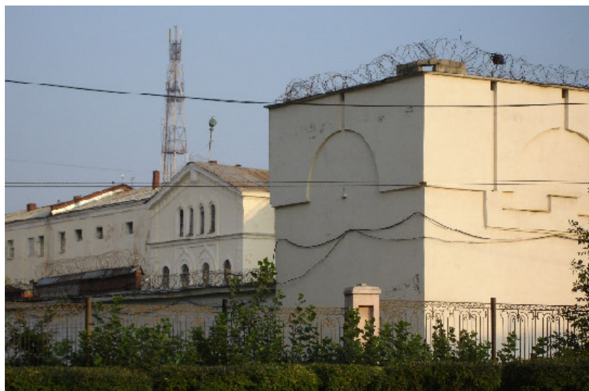
The detention Centre in Yekaterinburg code-named UshCh 349/2 or IK-2 in Russian, where detainees are reportedly routinely tortured. ©AI
